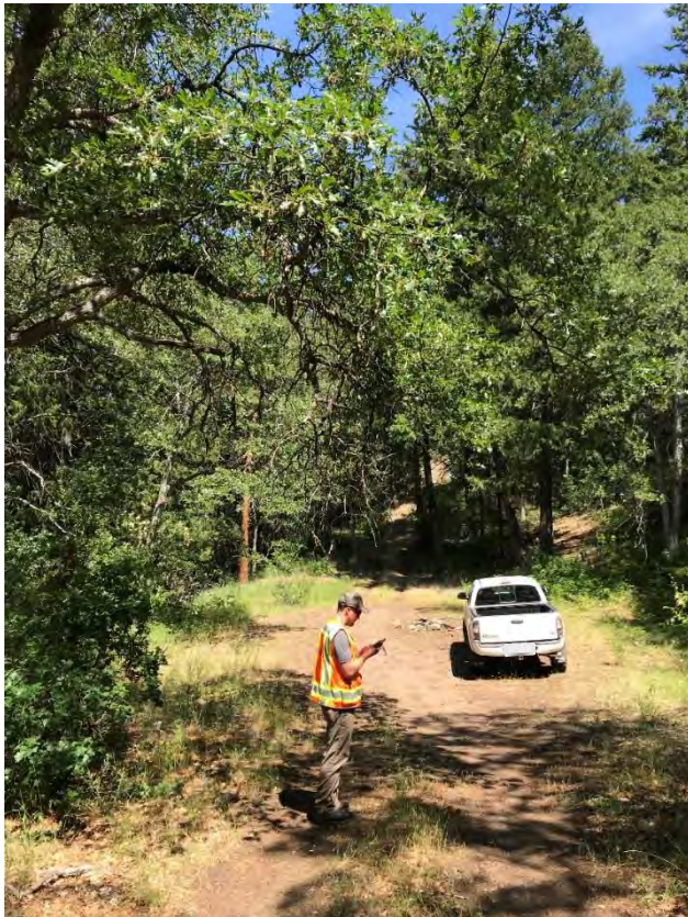
Photograph 17. ARM 9 – Oak tree limb would be removed for crane access to LT-B4.
