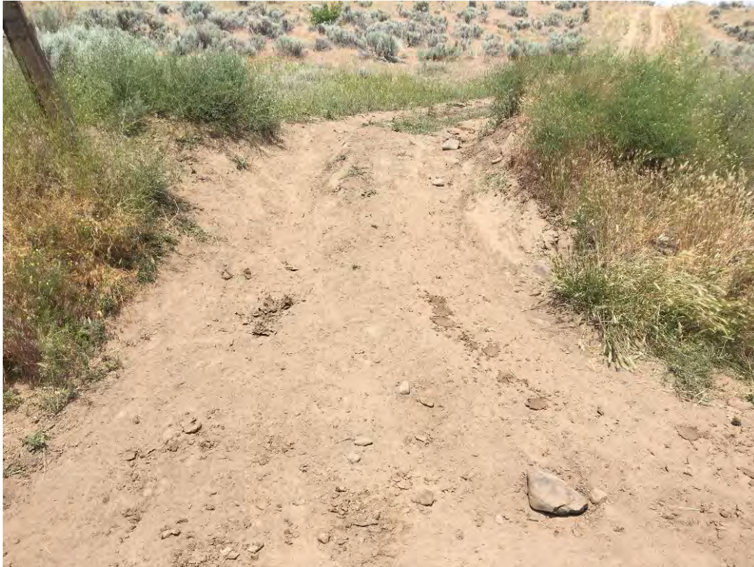
Photograph 7. ARM 1 - Roadside ditch adjacent to French Road would be filled to allow access to OB-2.
