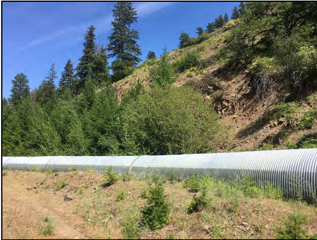
Photo 7: LT-B4 work area and associated habitat.
