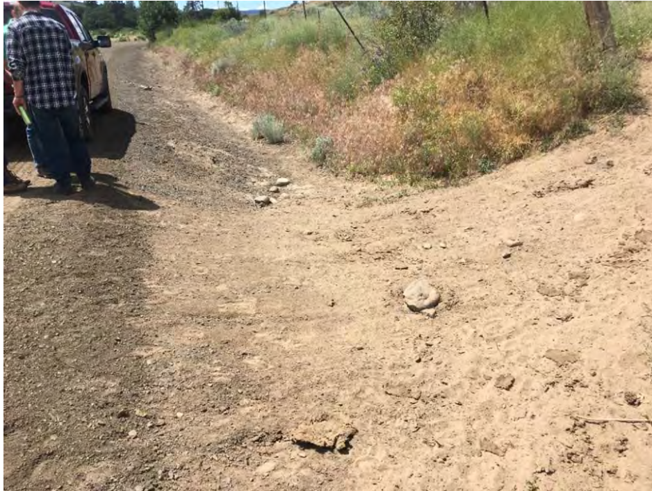
Photograph 3. At Access Road Modification (ARM) 1, the roadside ditch adjacent to French Road would be filled to allow access to OB-2.
