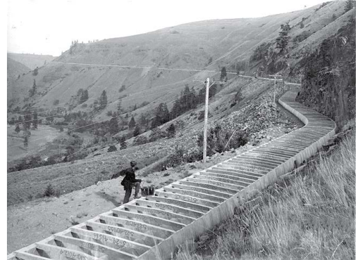
Photo 1, Main Canal, circa 1910. The canal was constructed from precast concrete segments.
