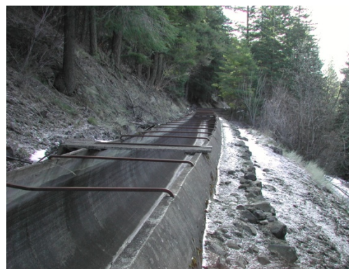
Photo 3, Typical Upper Main Canal Configuration and Topography, 2013.
