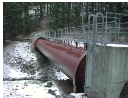
Photo 4, Typical 102-inch-diameter pipe bridge at drainage crossings, 2013.
