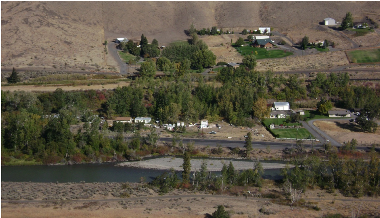
Figure 4-1. View of Site 3 for the WCPS
