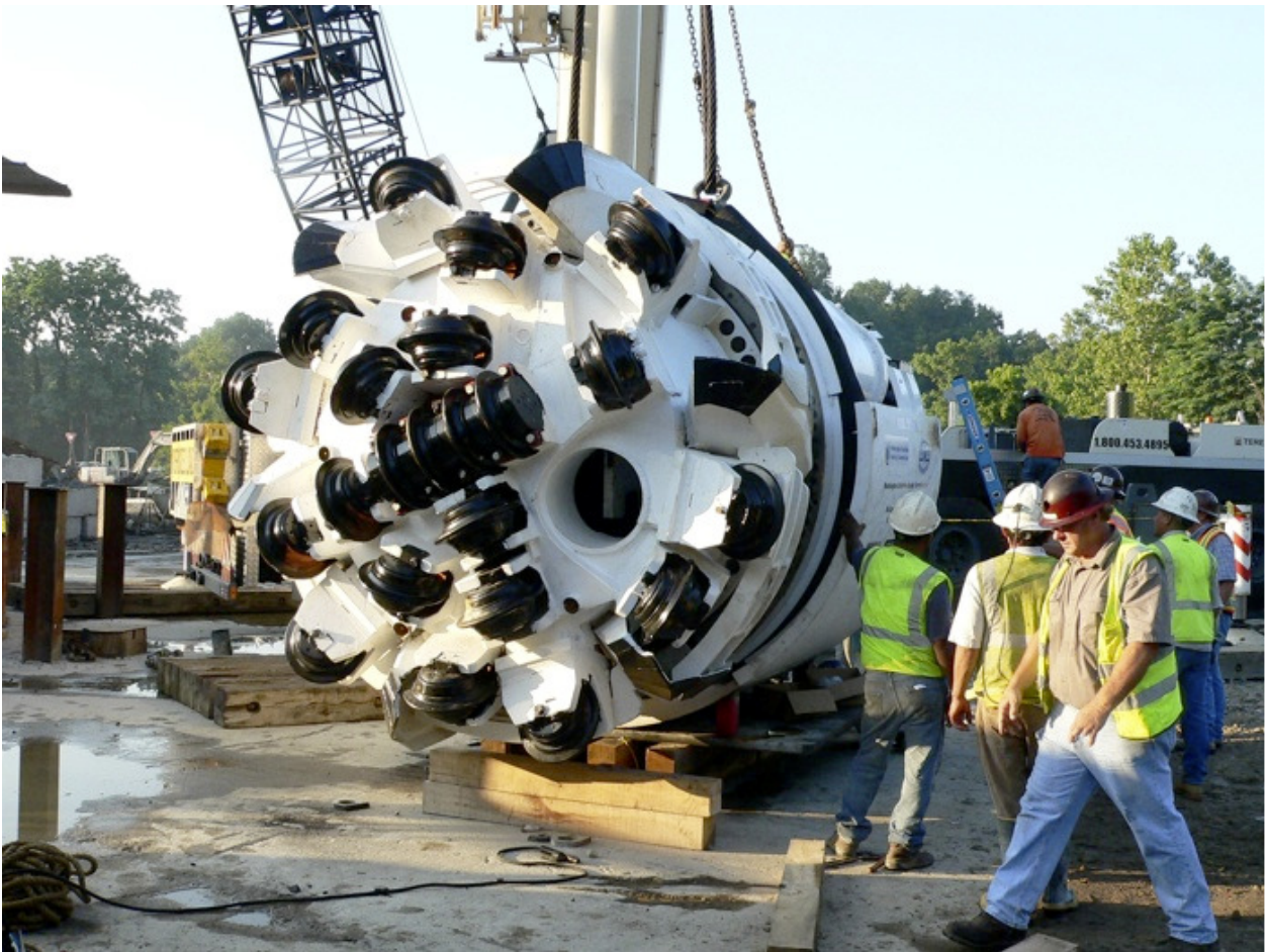
Figure 4-9. Main Beam Gripper TBM Cutting Head (10 foot diameter)
