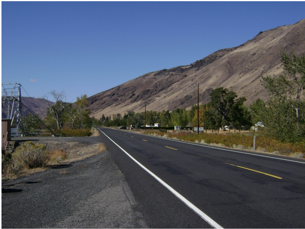
Figure 4-7. Highway 12, Looking West
