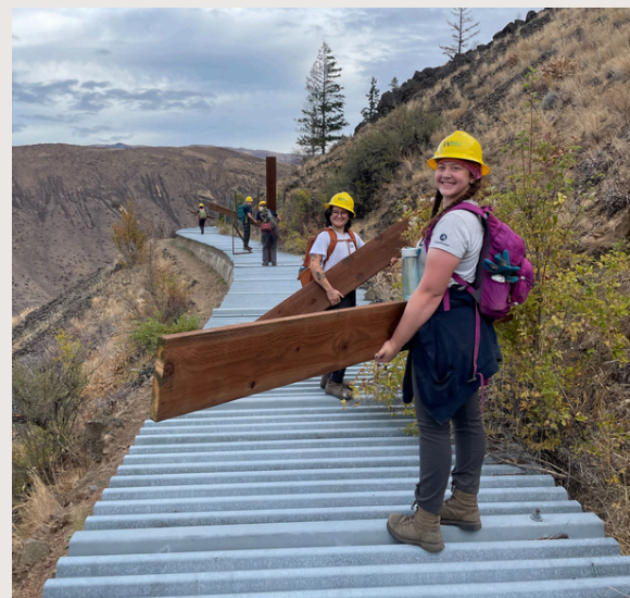
WCC crews staging materials for wildlife crossings.
