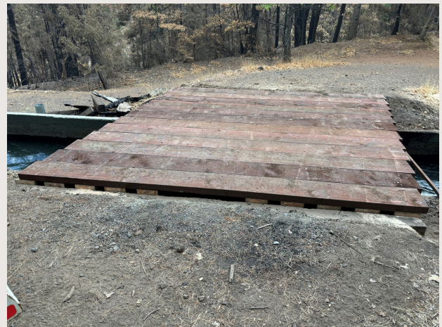
After: Bridge rebuilt by district crews.
