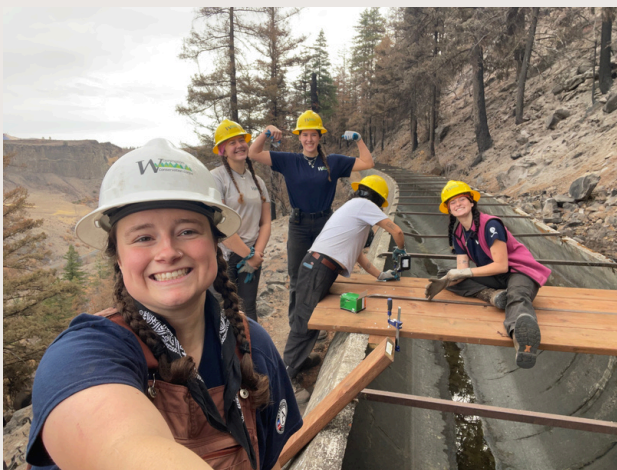
Washington Conservation Corps (WCC) crews completing wildlife crossings.
