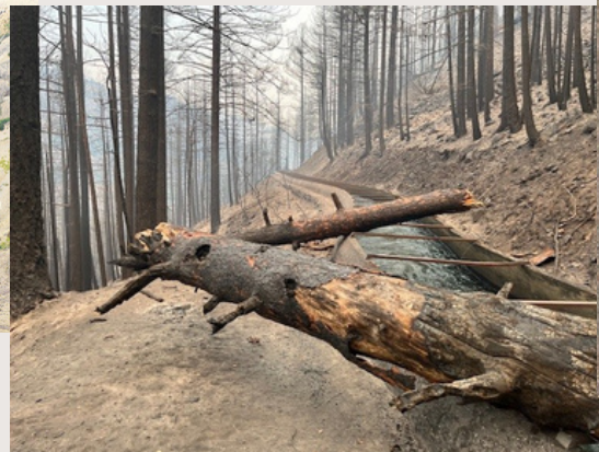
Before: Burned trees fall on top and into canal posing serious risk of catastrophic failure. Dozens have been removed but thousands of dead standing trees remain a threat.
